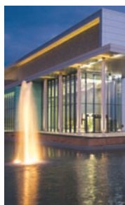
The new Manufacturing Technology Centre near Coventry.
